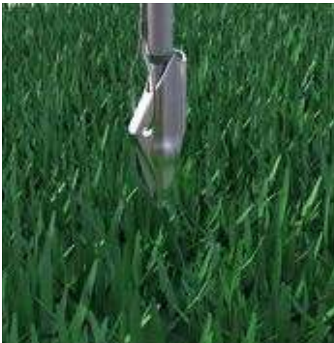
Anchor 3 being driven into the ground.
